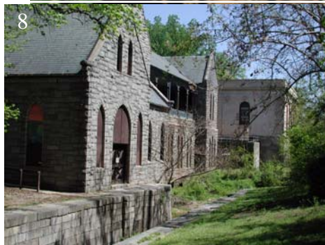
7. The River 8. The Pump house
